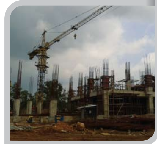
BASIC INFRASTRUCTURE DEVELOPMENT: INTERNAL ROADS, WATER SUPPLY & SUB-STATION WORKS IN PROGRESS
